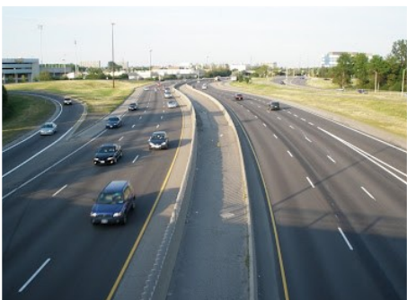
The highway's profile was designed to have wide landscaped verges and a grassy median. It was actually built that way, with shoulder-less lanes, a wide green median strip, and a concrete roadbed. This shot is from the early 1960s looking west towards the Alta Vista overpass. Looking east today from the same overpass, the greenery has been sacrificed for another travel lane and the grass strip is long gone.
