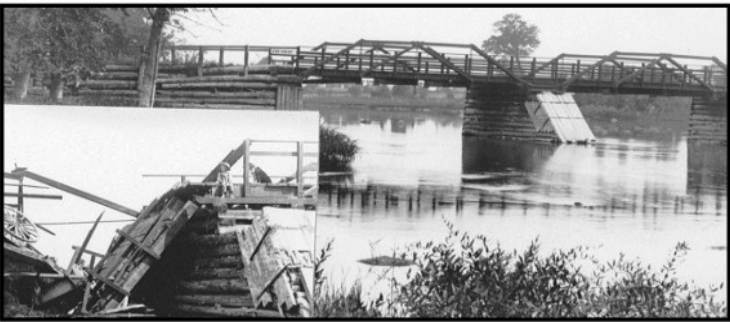
Hurdman Bridge Span collapse (c. 1902)
