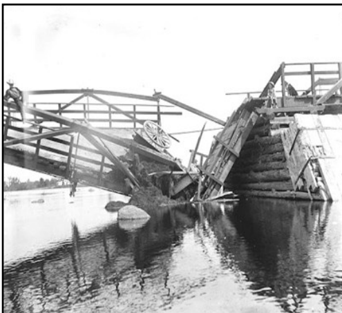
LEFT: A broken span on Hurdman's Bridge, July 29, 1902.
