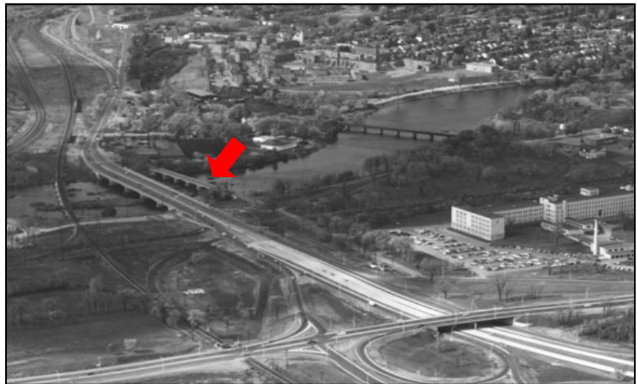
ABOVE: Hurdman's Bridge to the right (north) of the "new", large Queensway Bridge, 1958
