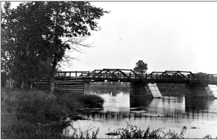
ABOVE: The first Hurdman's Bridge, c 1875
